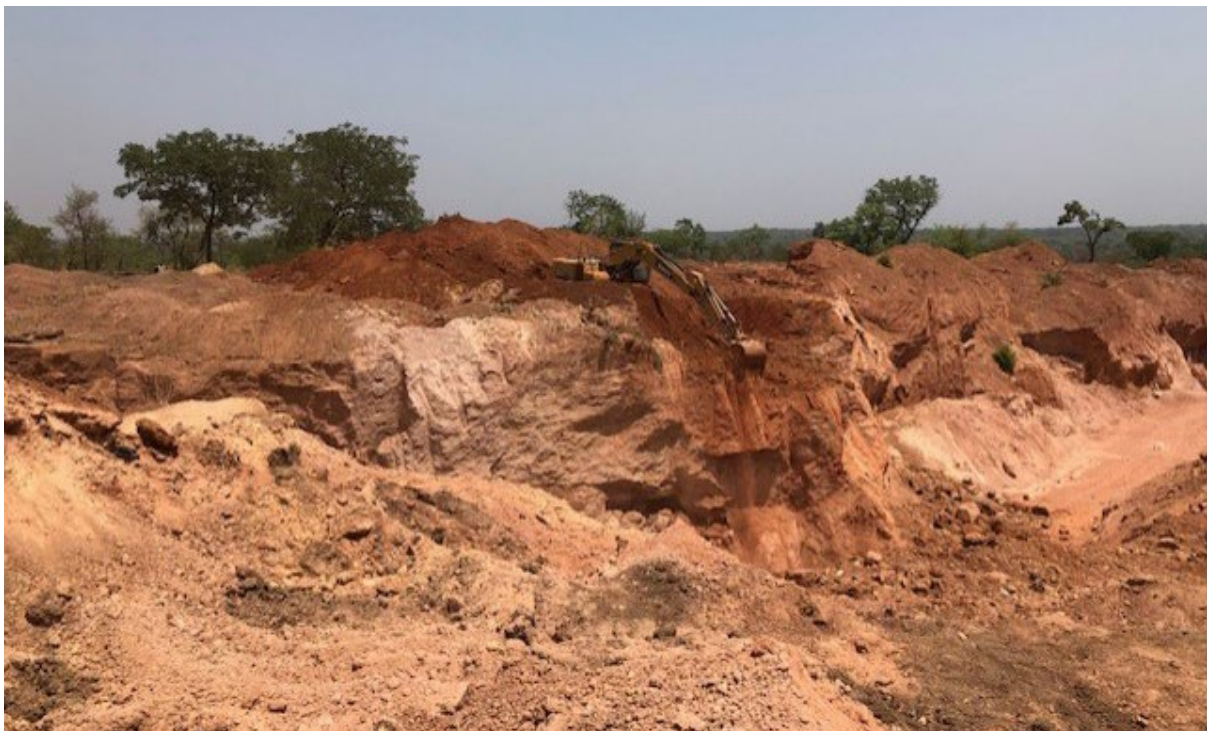
FIGURE 4. An excavator used in ASM in Guinea
